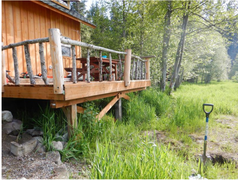
Photograph 3: Large deck will be removed as part of the Reasonable Use Exception project
